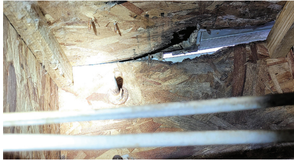
Inside basement upward view of failed sheathing and flooring underneath door
