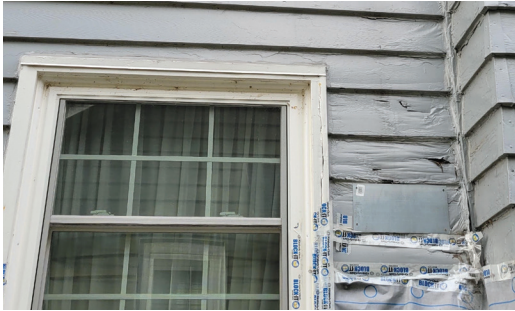
Damage from water and ice penetration since added addition
