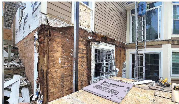
Hidden water damage behind siding and door edges for last 22 yrs.
