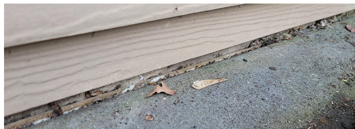
Improperly installed ledger flashing for a deck
